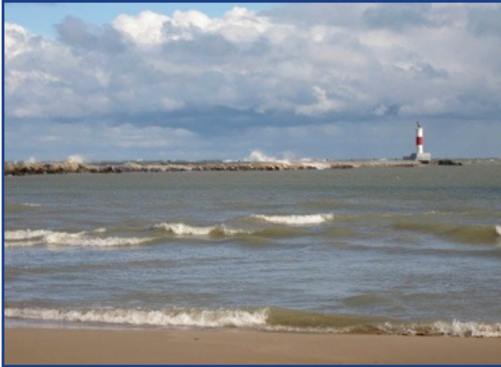
Harbor at Waukegan, Illinois Credit: Elva Busch
